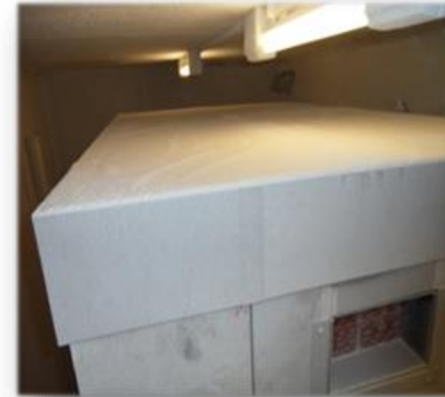
...dust deposits after the test ...
